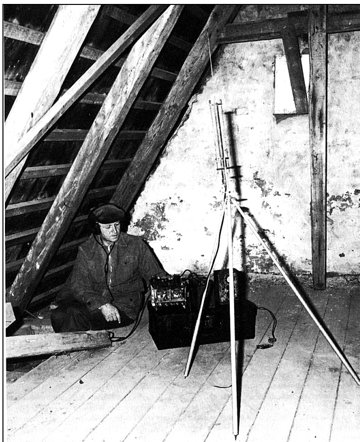
A reconstruction. Ole Moeller Jensen from Herning in tower of Rind Church south of Herning working with the 'Eureka' transmitter used for sending navigating bearing signals to RAF/SOE weapon planes.
